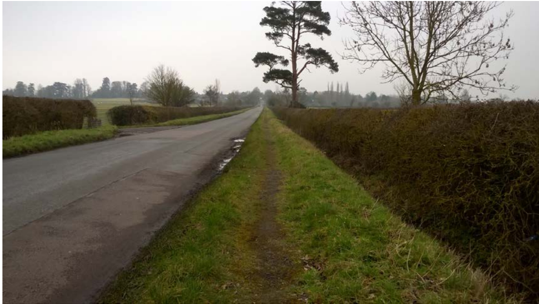
New Road – grassed over surface from A413
